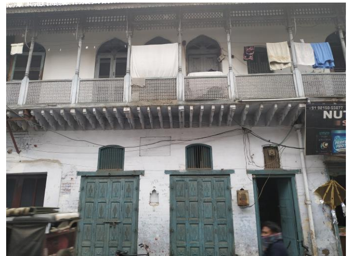
Figure 1. View of a shop-cum-house in Sadar Bazaar area, Karnal
