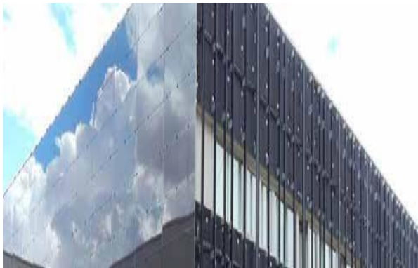
Figure.3. Application of BIPV as a curtain wall for a building.
