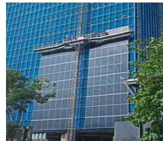
Figure.1. Data centre at Mumbai with BIPV
