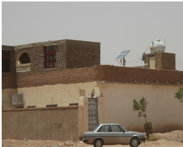
Fig.2 Module Placing on Top of the House's Roof at Alazhari City
