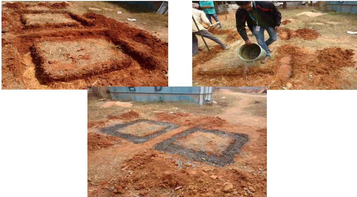
Fig. 7 - Excavation and concreting for the foundation of size 1.5m x1.5m
