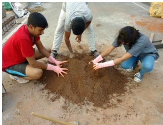
Fig. 3 – Mixing of soil, sand and cement uniformly
