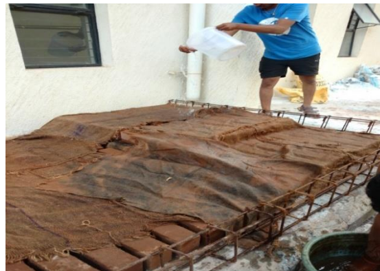
Fig. 6 - Curing of blocks
