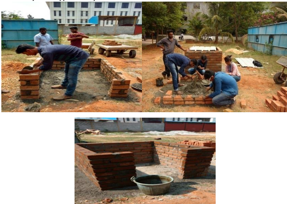
Fig. 8 – Construction of masonry wall of size 1.5m x1.5m x 1.5m
