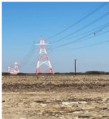
Figure 7. 132 kV Double conductor two circuits of Line 2
