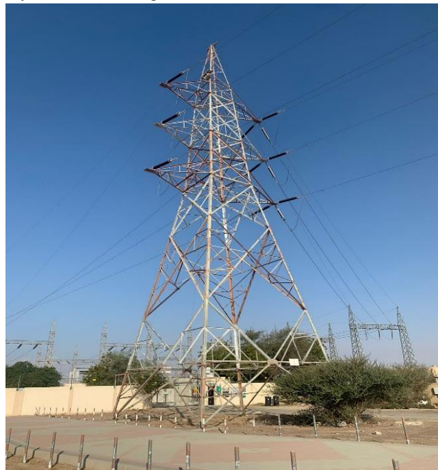
Figure 8. 132 kV Double conductor two circuits of Line 3
