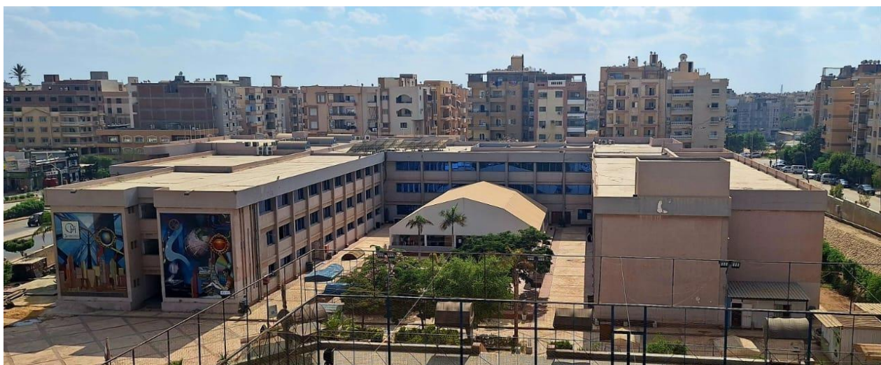
Fig (2) shows the building of the October High Institute for Engineering and Technology, indicating the location of the classrooms in the university buildings under study.
