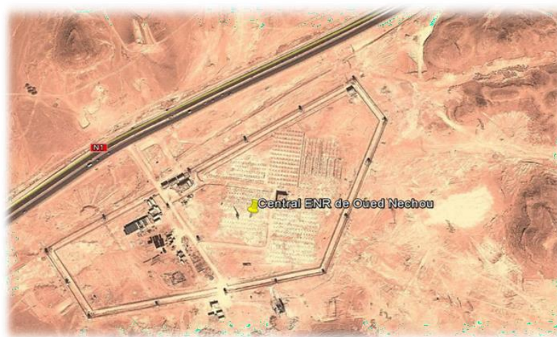
Fig. 1. Geographical location of the photovoltaic power plants 1.1MWp OUED-NECHOU, Ghardaïa City.
