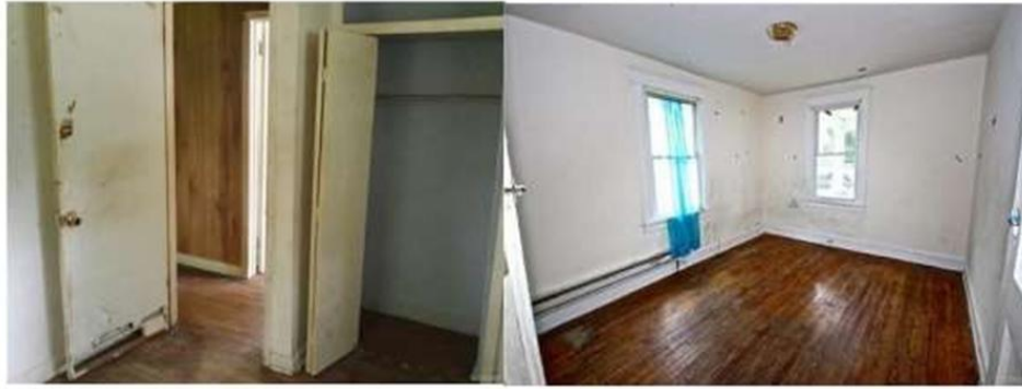
Figure 3: Room condition is critical, door damage critical, floor damage is major, b: Room condition is major, wall scuff moderate, floor damage major.
